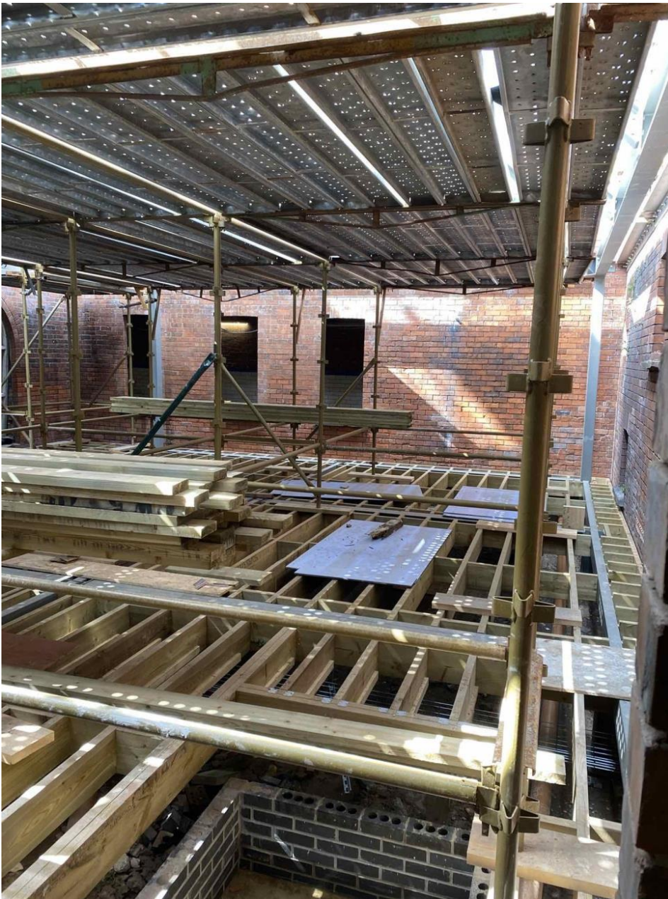
Fig 5- Templemore- existing courtyard area being roofed and floored to incorporate new café area
