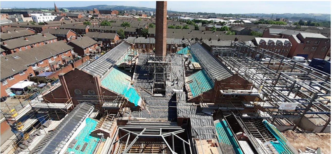
Fig 4- Templemore- new lantern style glazed roofs to main pool, derelict pool and slipper baths (steel frame for new building to the right-hand side)
